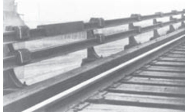
Typical Double Rail Installation
