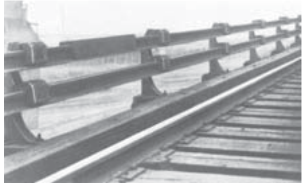
Typical Double Rail Installation
