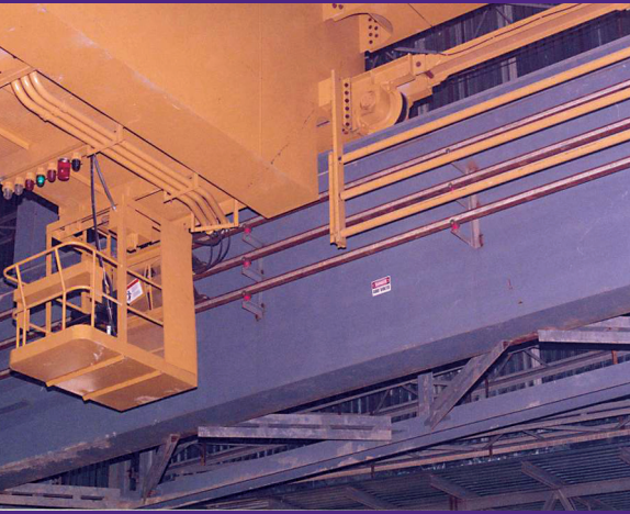
80" Roll Processing Crane
