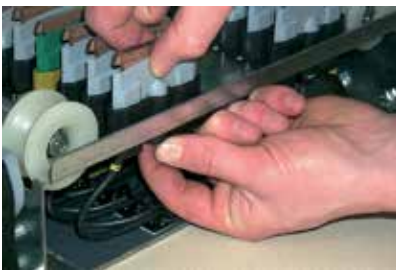
Replacing the carbon brushes.
